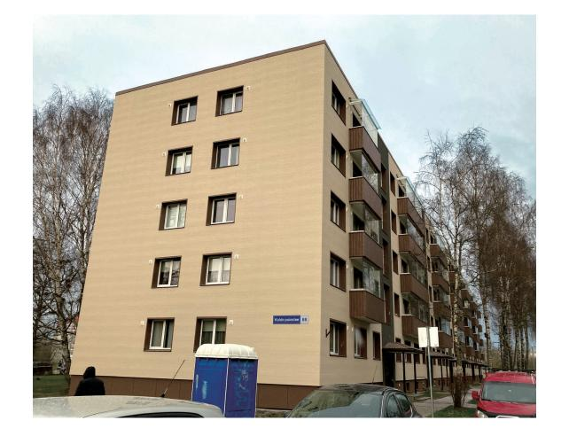
Four-side Tongue and Groove By using 1,820mm panels, it is possible to create a neat and beautiful wall surface with inconspicuous seams.
